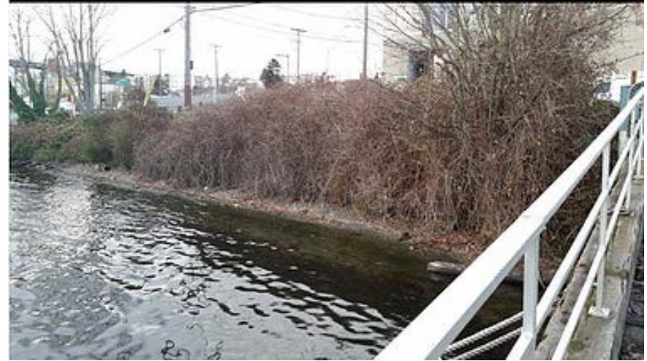
Waterway 22 is located at the corner of N Northlake Way and Stone Way N
